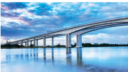
Monitor infrastructural deterioration in bridges
